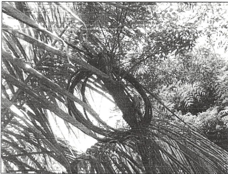
Plate 5 Improper alignment of gas pipe in Raichur
